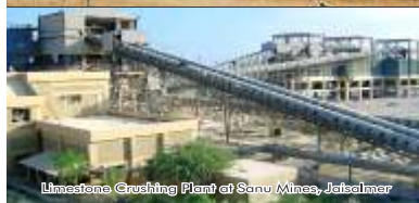
Limestone Crushing Plant of Sanu Mines, Jaisalmer
