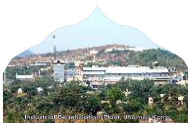
Industrial Beneficiation Plant, Jhama, Kota
