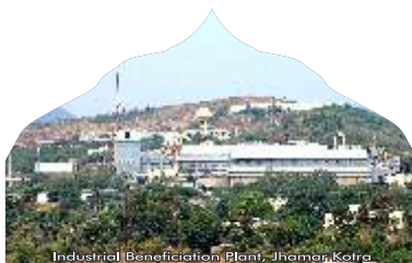
Industrial Beneficiation Plant, Jhama, Kota
