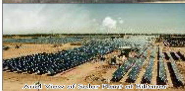
Aerial View of Solar Plant at Bikaner
